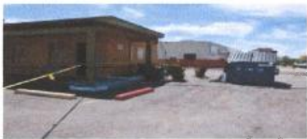
5. Western view of motel & dumpster
