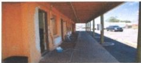
3. Bow & Arrow Lodge, south to north view, truck in front of room 27
