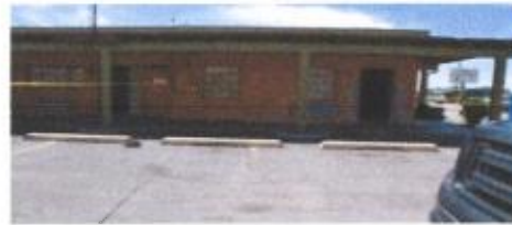
6. Room 27 at northwest corner
